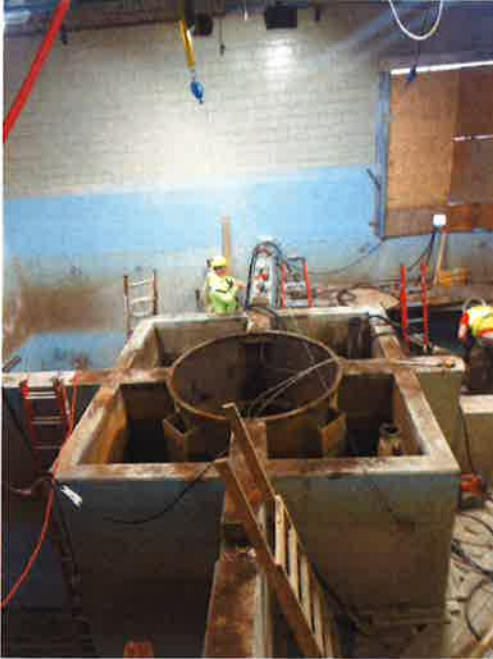
Demolition of existing filter structure.
