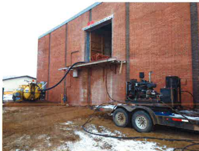
New door opening in existing filter area.
