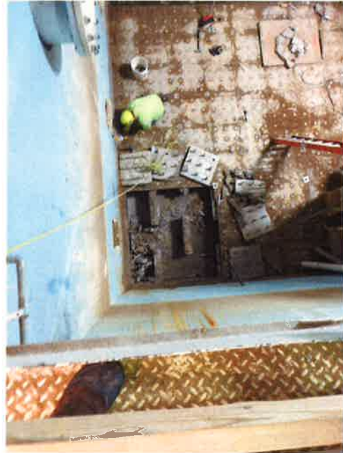
Demolition of existing filter underdrains.
