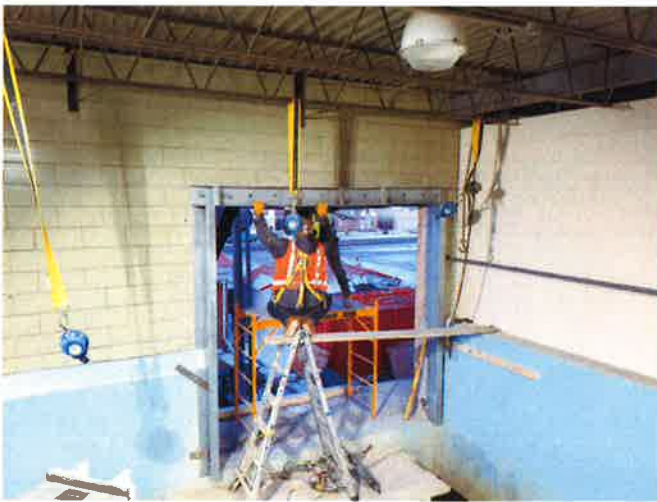
Constructing new door in existing filter area.
