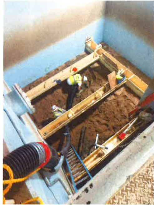
Removing existing filter media.
