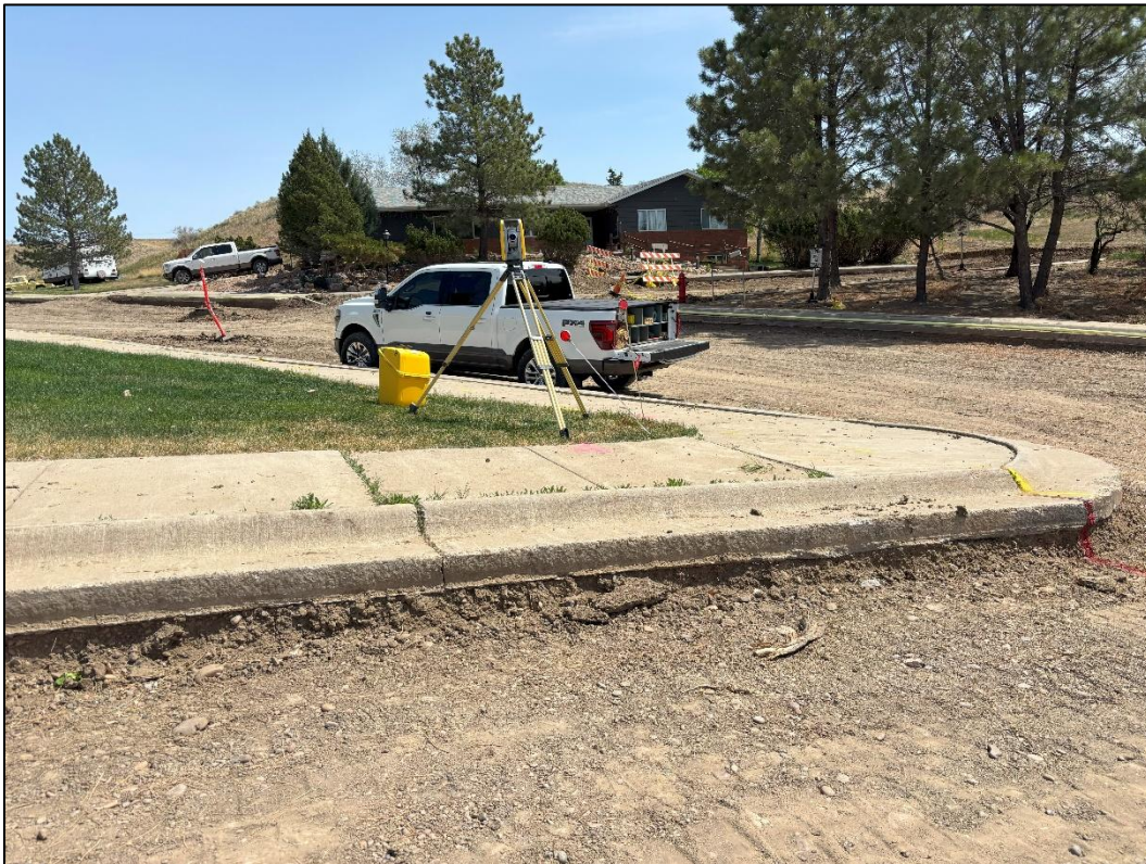
Figure 1: Surveying and staking.
