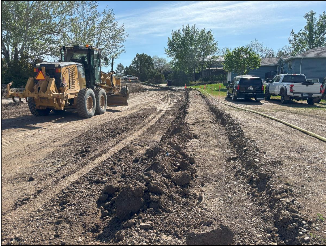
Figure 2: Preparing for sidewalk forming.
