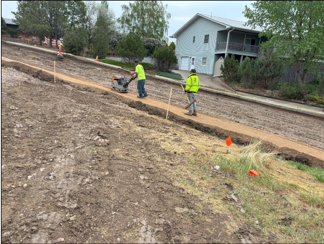
Figure 4: Compacting AB material placed under sidewalk.
