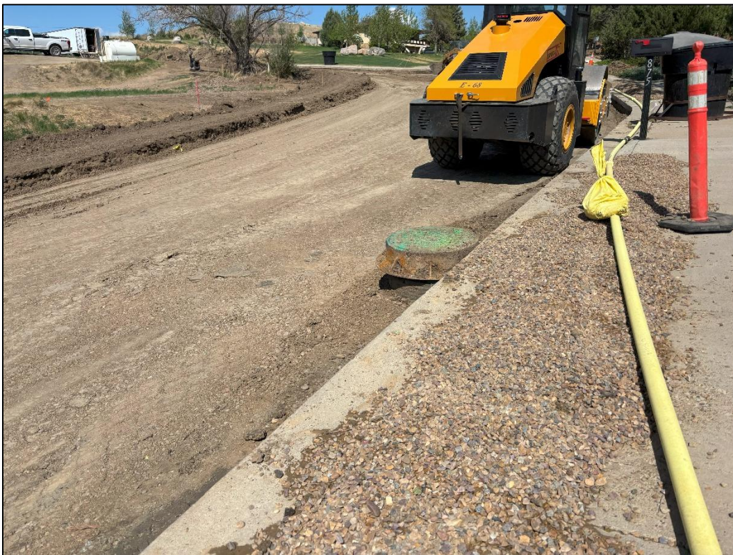
Figure 3: Compacting AB Material under road.
