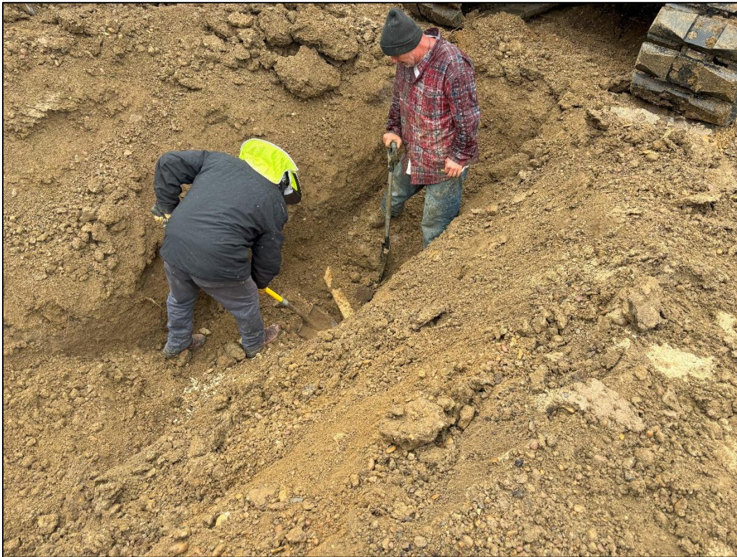
Figure 2: Connection of water service line.
