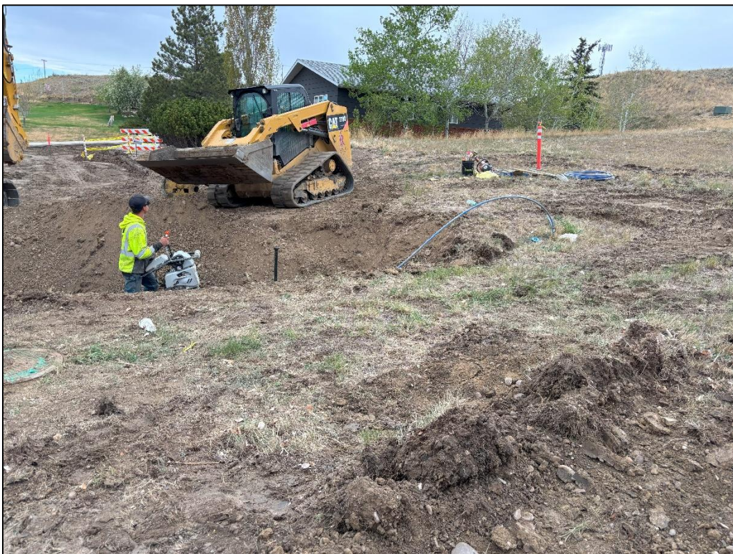
Figure 2: Connection of water service line.
