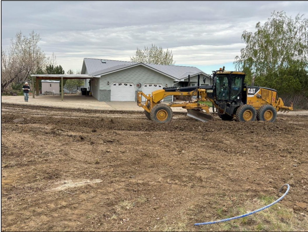
Figure 4: Grading Hall Terrace.
