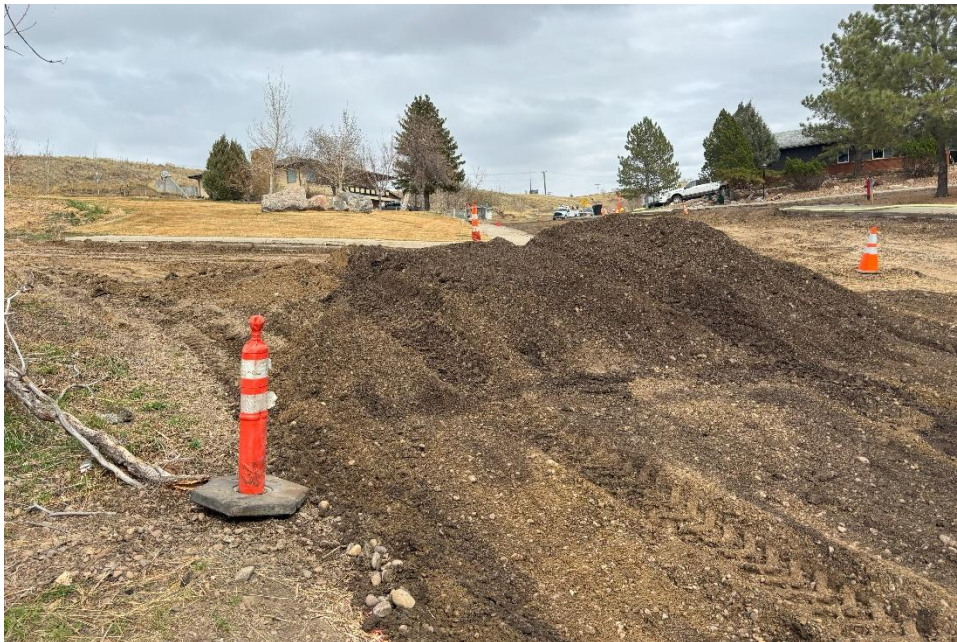
Figure 4: Remove 14" of topsoil.
