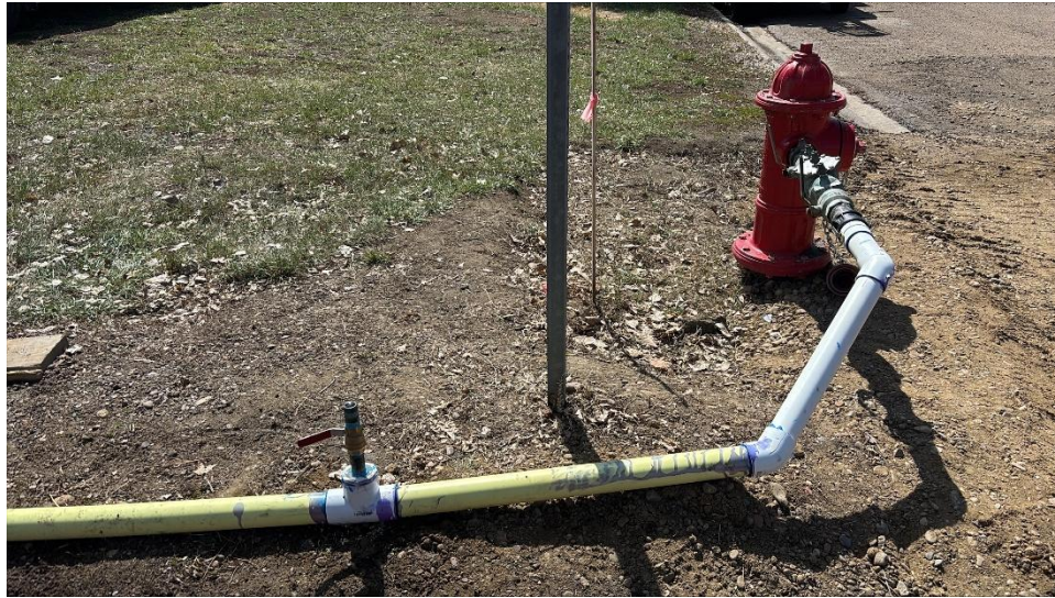
Figure 1: Installing temporary water piping.
