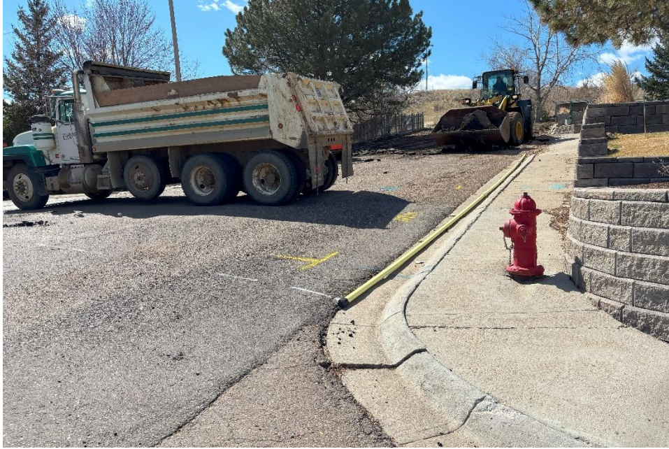
Figure 3: Removed remaining asphalt on Hall Terrace.
