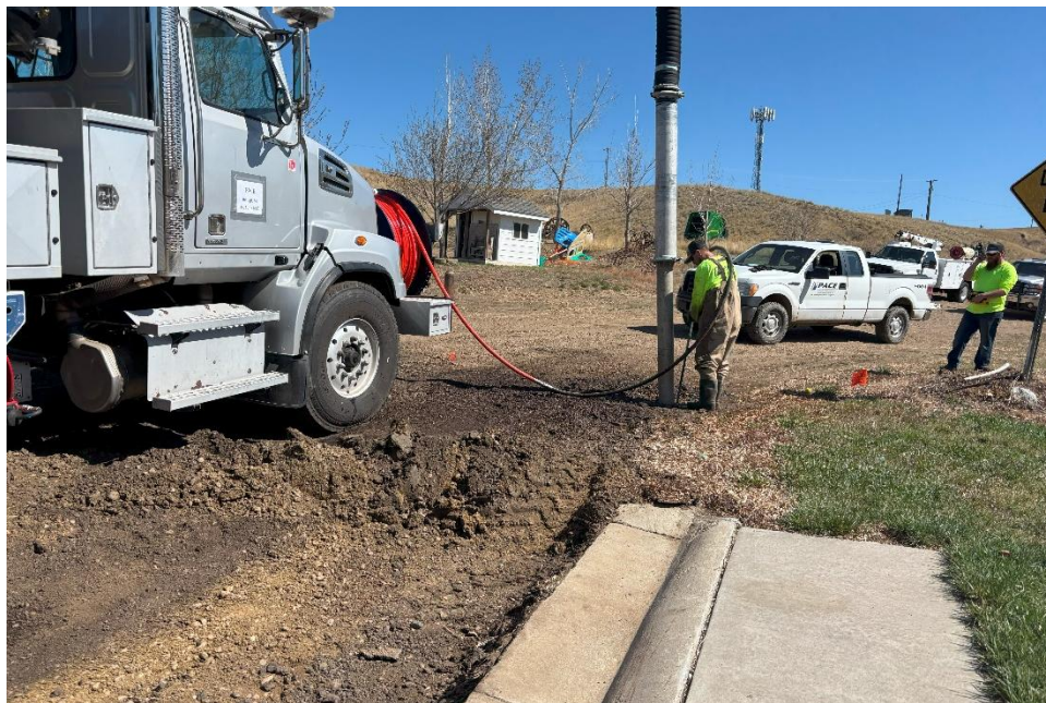
Figure 2: Located utilities with Hydrovac.
