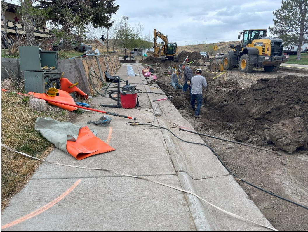
Figure 2: Repairing electrical line on East end on Hurley Drive.
