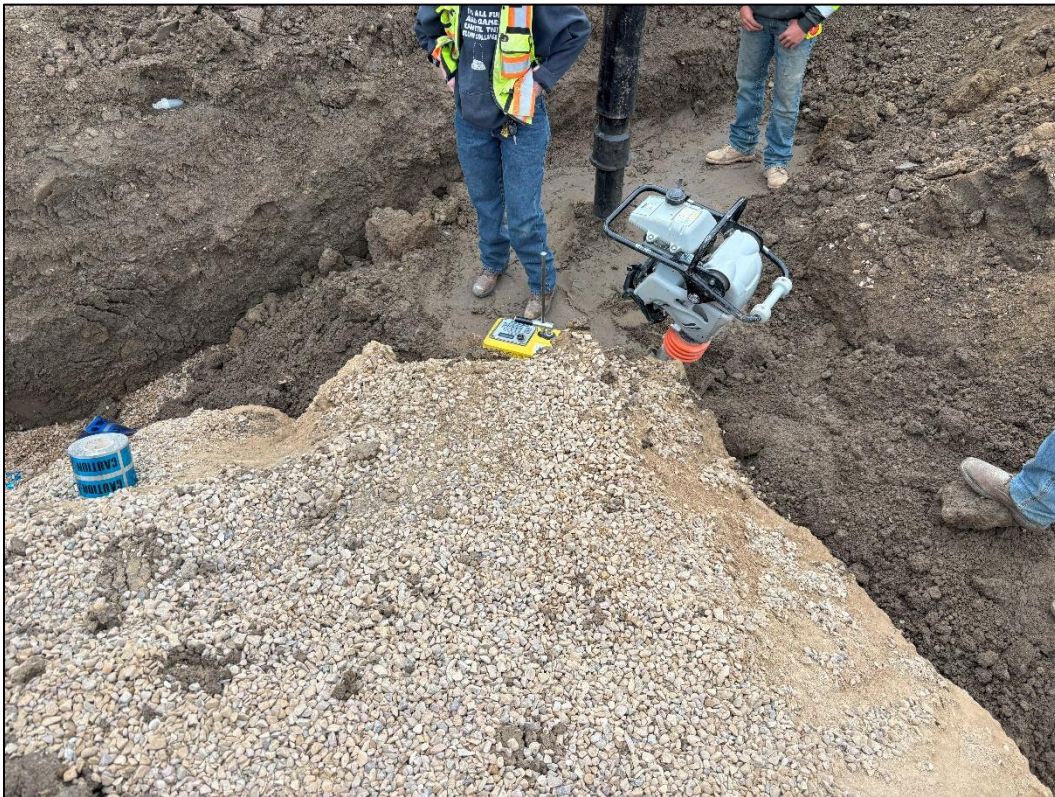
Figure 3: Density testing on Hurly Drive.
