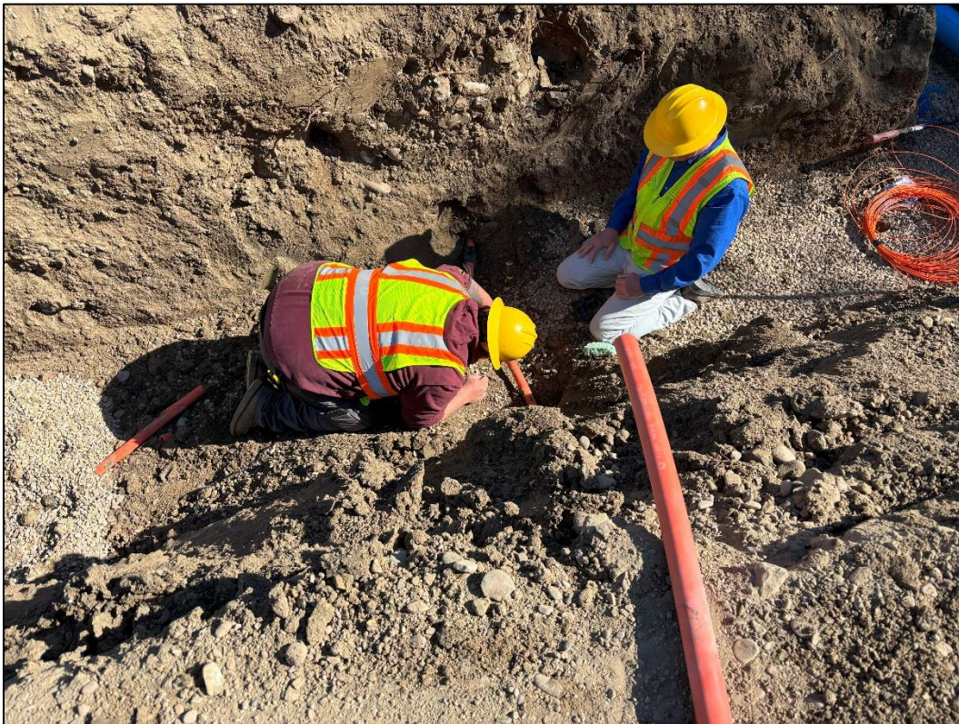
Figure 5: Repairing Fiber optic line near station 6+10.
