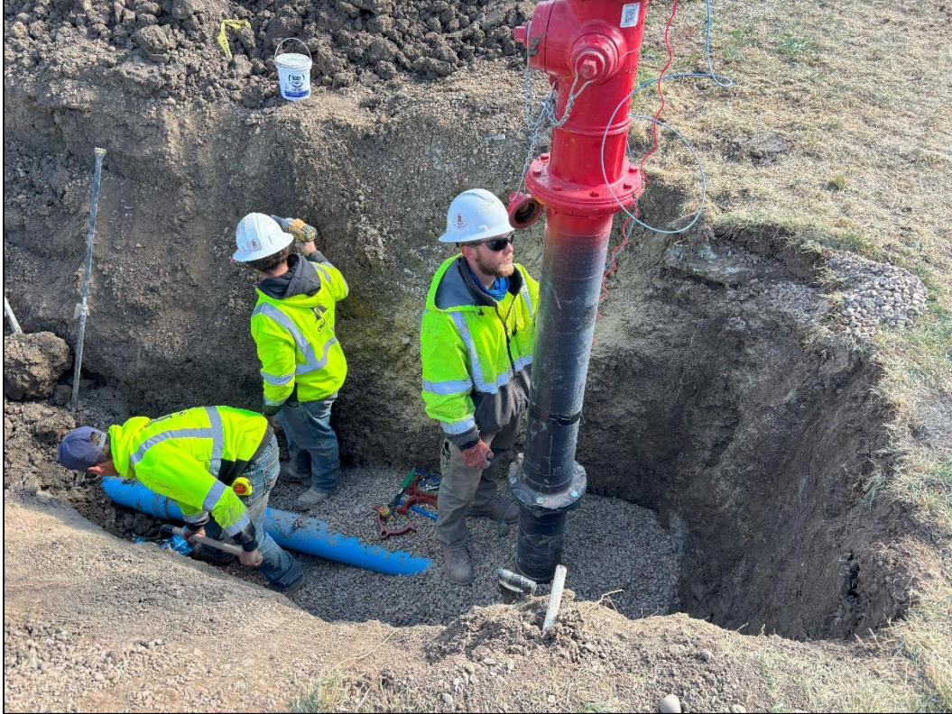
Figure 4: Fire Hydrant installed on Hall Terrace.
