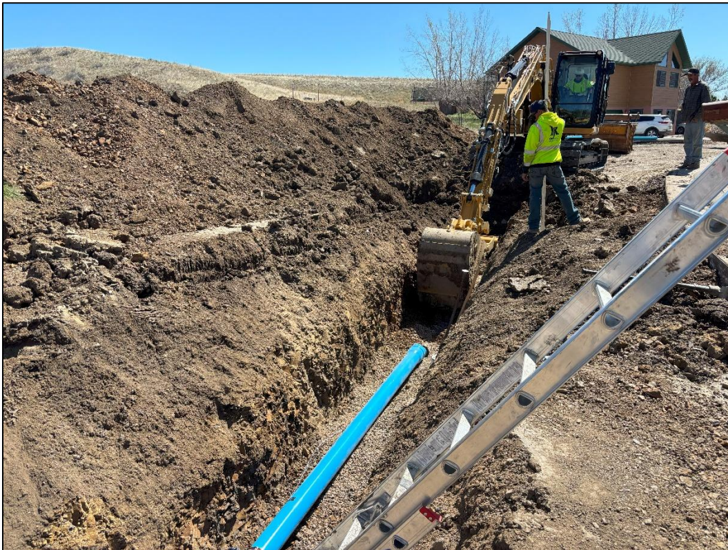
Figure 1: Water main trenching in Hall Terrace.
