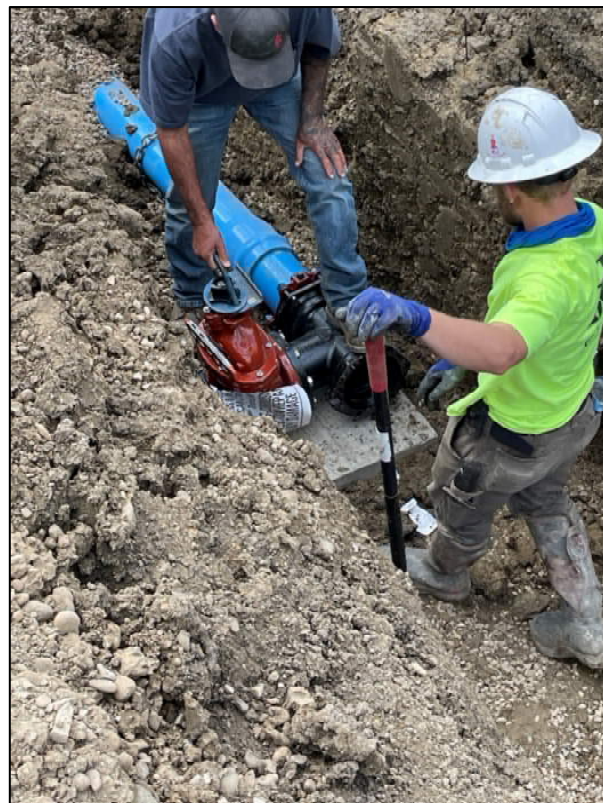
Figure 10: Installation of Gate Valve – intersection of Hurly Drive and Hall Terrace
