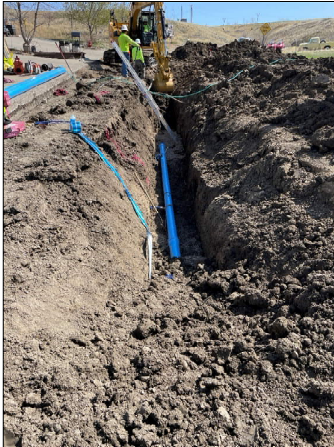
Figure 12: Water main installation – east end of Hurly Drive
