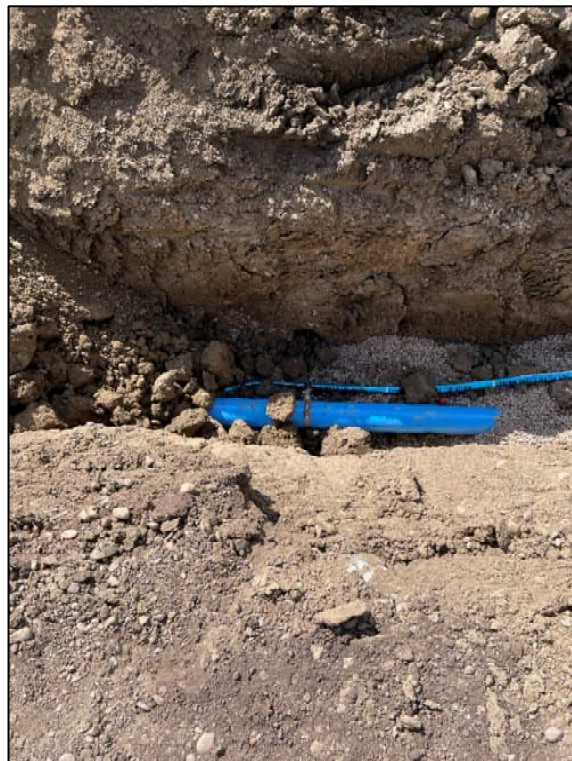
Figure 6: Water Service Saddle
