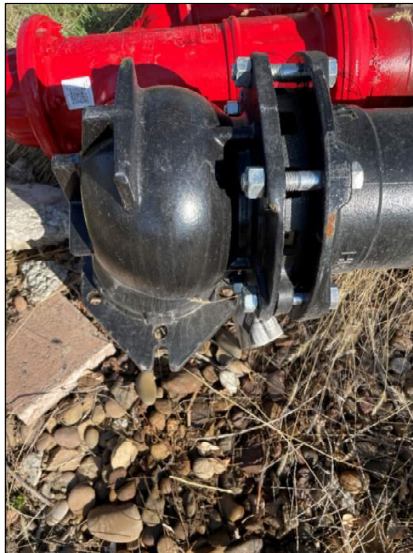
Figure 4: Fire Hydrant (boot) to be installed
