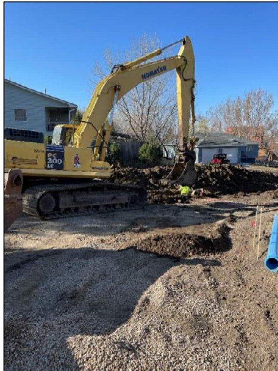
Figure 1: Water main trenching in Hurley Drive
