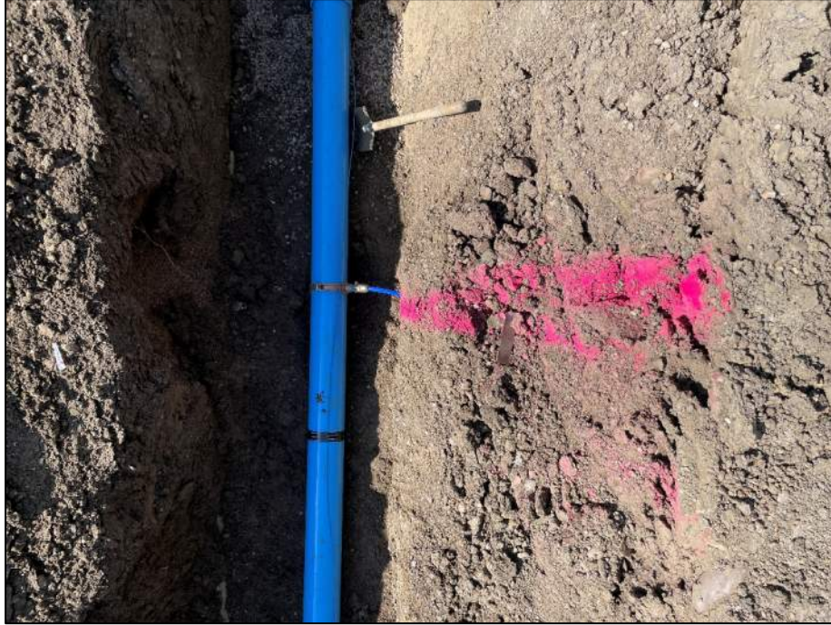
Figure 11: Water Service Connection for 726 Hurly Drive
